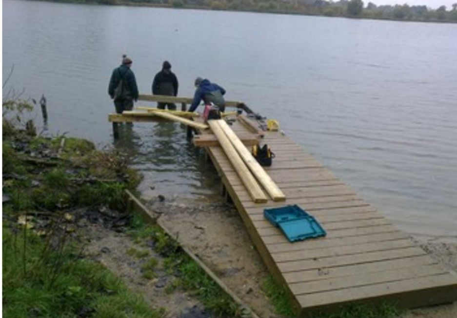
Sam, Peter and Ross working on the jetty
